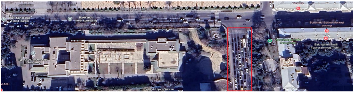
Fig. 1. Satellite image of one of the Bakikhanov Street intersections.
